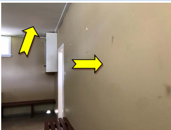
Photo 11. Interior, home change room, walls and ceiling – suspected lead-containing dark yellow and white upper coloured paint systems.
