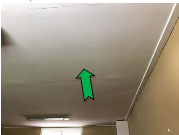
Photo 5. Interior, home change room, ceiling – non asbestos-containing fibre cement sheeting.
