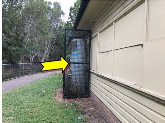
Photo 8. Exterior, north elevation, hot water heater – suspected SMF internal insulation material.
