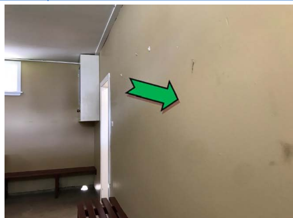
Photo 6. Interior, home change room, wall – assumed non asbestos-containing fibre cement sheeting.
